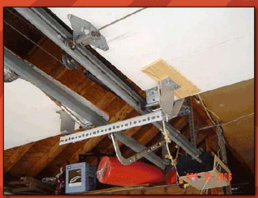
The homeowner of this house apparently did not want to buy two garage door openers and installed one in the center of the two doors and connected them.
