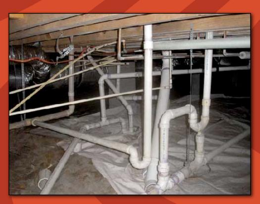
Wasn't there a screen saver like this? This is a picture of some amateur plumbing work for the drain system of a home.
