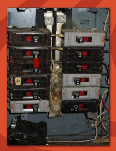
This is a photograph of a rat that entered an electrical panel through an open knockout. When it came in contact with the grounded box, it got fried! I show this picture, which I carry to all inspections, to homeowners who poohpooh my complaint of open knock-outs at electrical panels.
