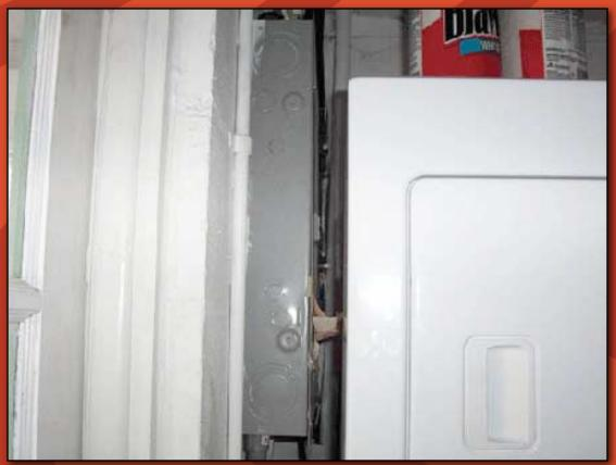
This is a picture of an electrical panel with an apartment-size washer/dryer combo sitting right in front of it. Hope the owners don't have to get into it in a hurry in case of an emergency.
