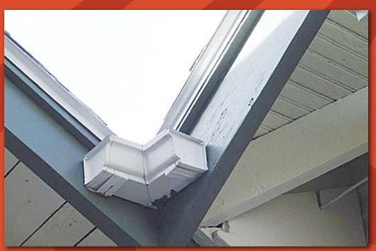
I found this rain gutter capped on both ends. I wasn't surprised to find decayed material inside.
