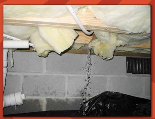
I captured this photo in the crawl space of a new-construction home after it had passed all municipal inspections. The bathtub drain was never completed.
