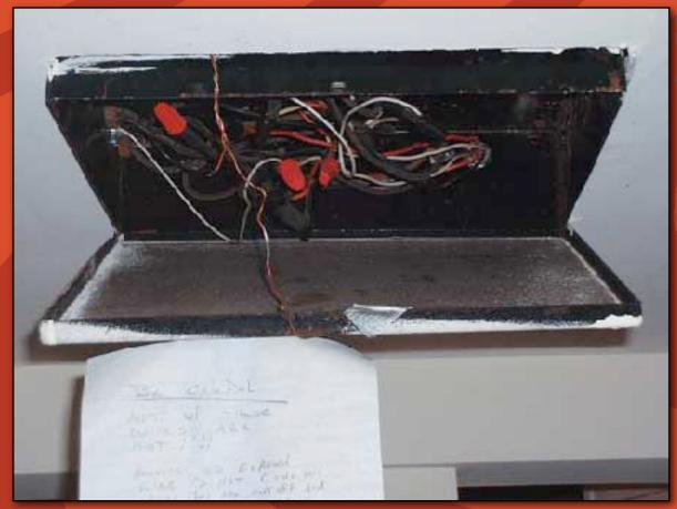
I guess we would call it a 1921 oversized junction box (1' x 1.5')! Someone left a note attached indicating some of the wires were hot!! This 'box' was located on the basement ceiling and open when I found it!
